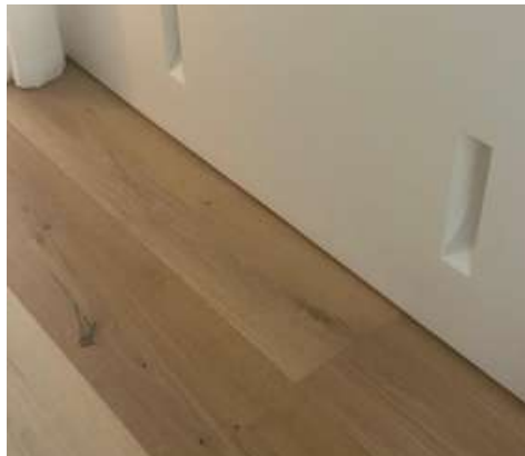
Skirting boards: Inset detail.
