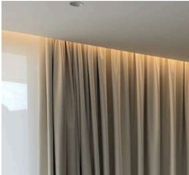
Recessed for curtain rods.
